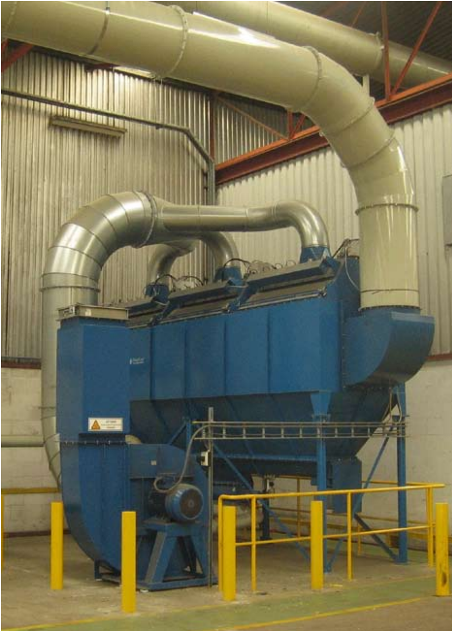
PowerCore® dust collection unit with a capacity of 20 000 m³/h at the Isover plant
