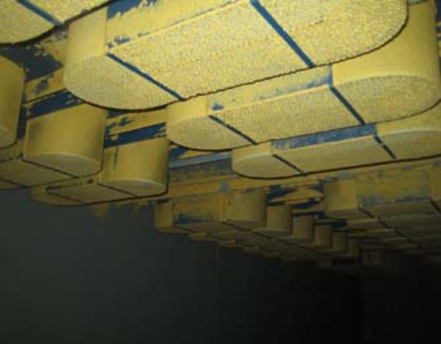
5 The dirty air side of the PowerCore® unit. Bridging between the filters and resultant plugging are successfully avoided
