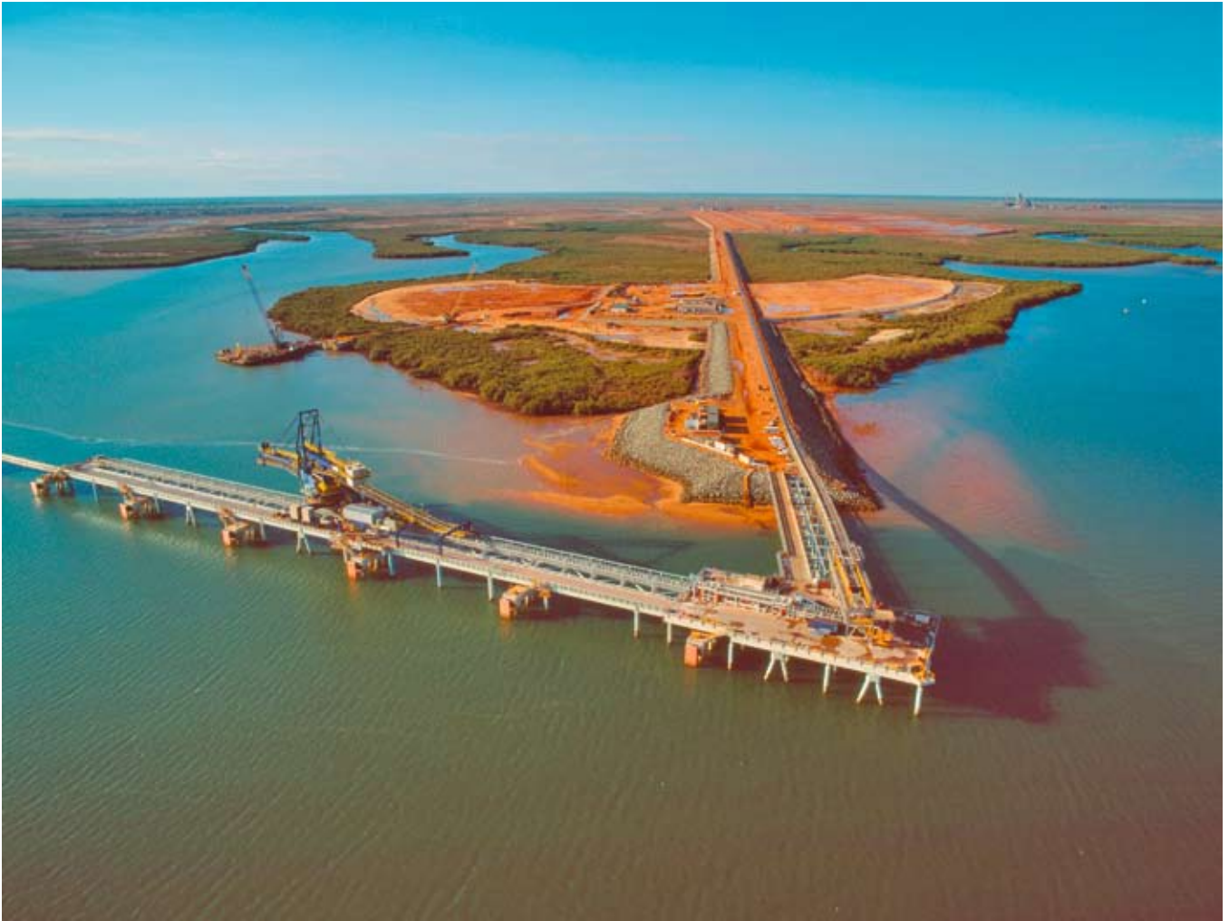
Anderson Port for iron ore (Fortescue)
