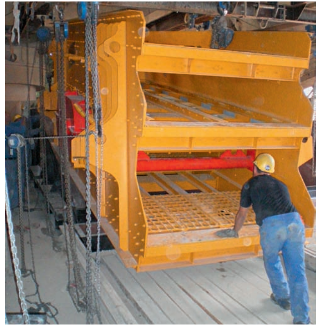
5 Installation of a screen in the same position in changed surroundings
